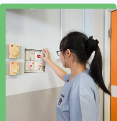
Kennix switching off the air conditioner.
